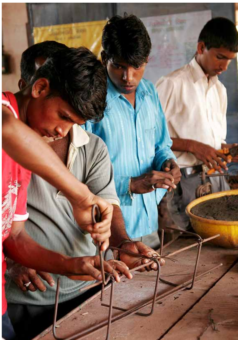
Students prepare metal frames for casting. Why can't all schools be run this way?
